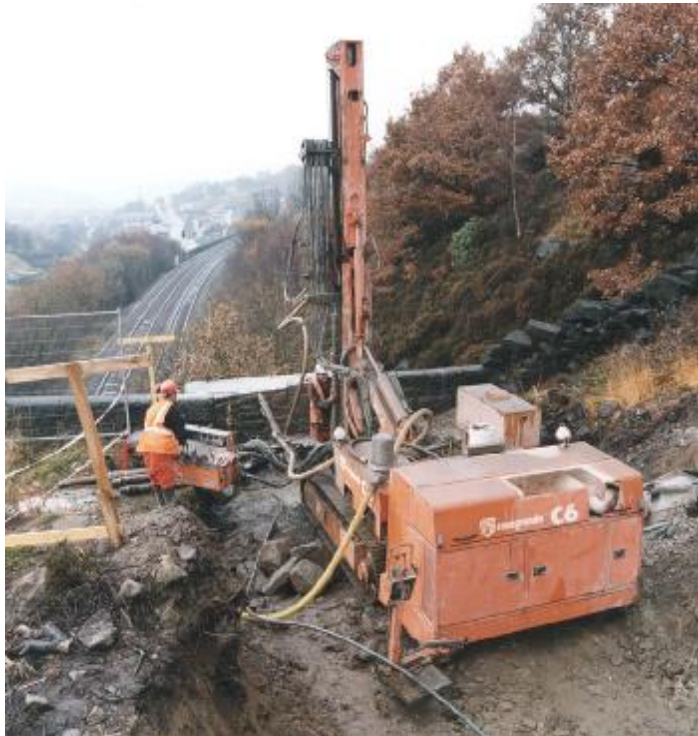
Figure 5 : Casagrande "C6" rig operating above the tunnel
