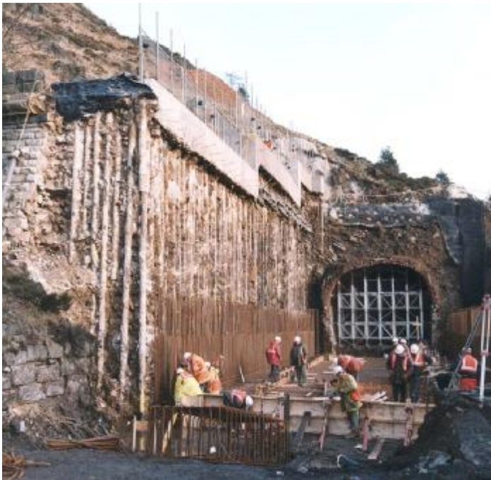
Figure 6: A view of the wall shortly after demolition of the tunnel
