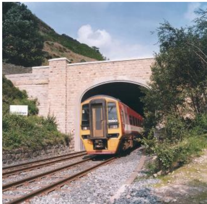
Figure 8 : The re-instated tunnel in operation
