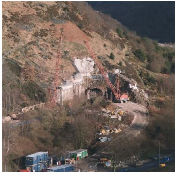
Figure 3 : A panoramic view of the site during construction
