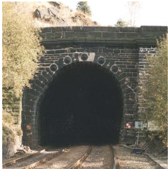
Figure 1: The west portal before the start of site works
