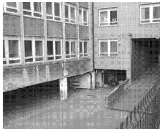
Fig. 7: Colmstock House – rear view
