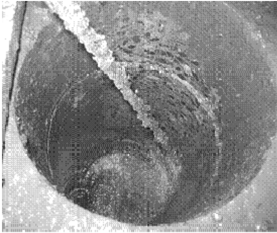
Fig. 3: Cleaning Ankerbond & core hole
