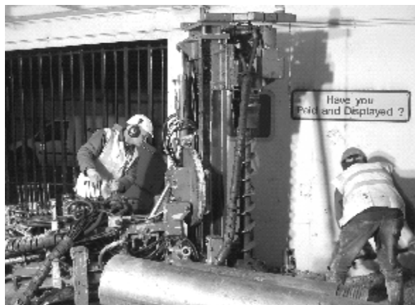
Fig. 17: Auger drilling minipiles
