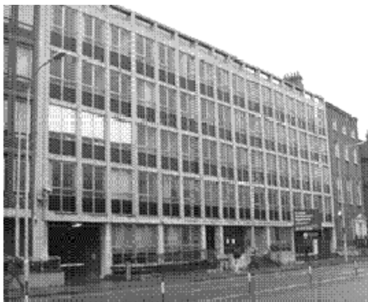
Fig. 6: Colmstock House – front view
