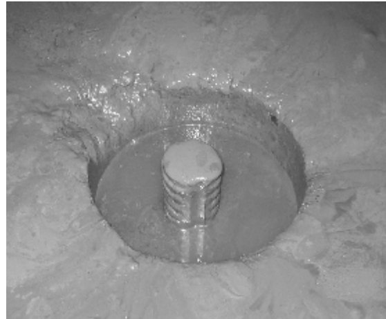
Fig. 4: Minipile ready for final topping up
